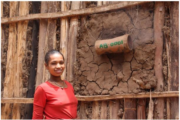
The outlet is ready to conduct the smoke through the wall out of the dwelling
