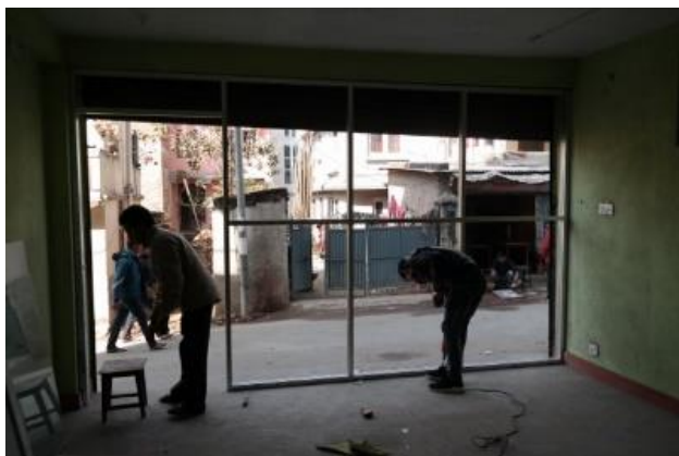
Interior fitting with separation to the street
