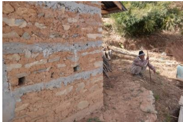
Earthquake-proof design with ring anchors
