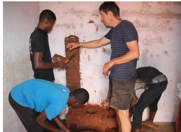
Chimney construction and lining the stove
