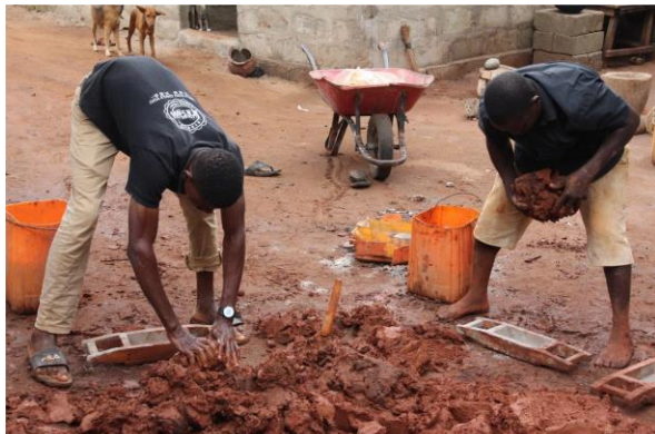
Filling the brick forms
