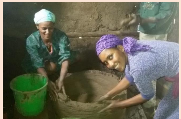
Genet and Yeshwa at pilot stove construction
