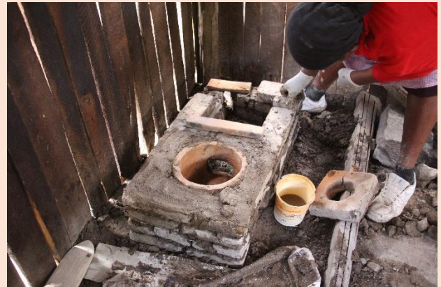
The Kenya stove in the shell - the clay insert is visible
