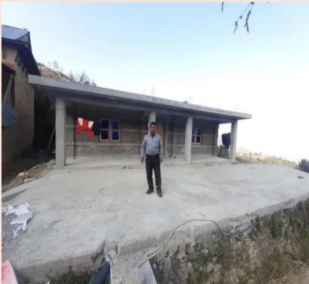
In front of the new earthquake proof house
