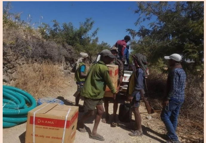
Delivery of tubes and the pump
