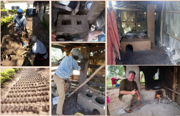
Preparation and production of bricks and building elements for the construction of the first stoves by the trained students (example: pottery school).
